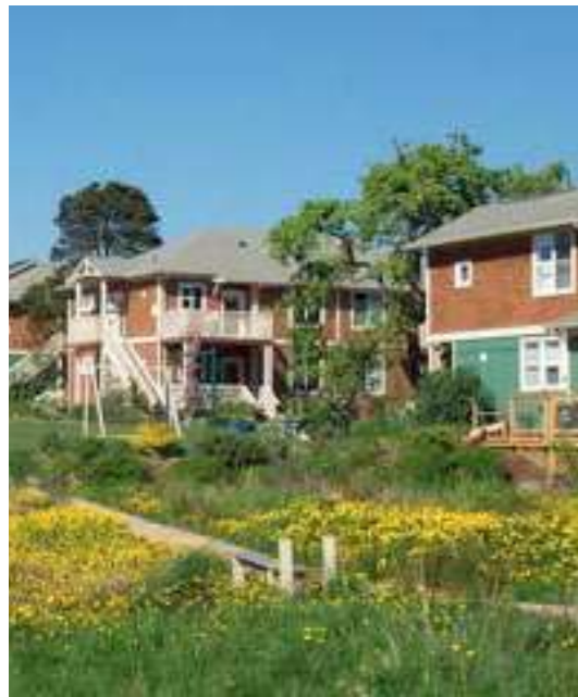
Co-housing development with detention basin. Canada.
