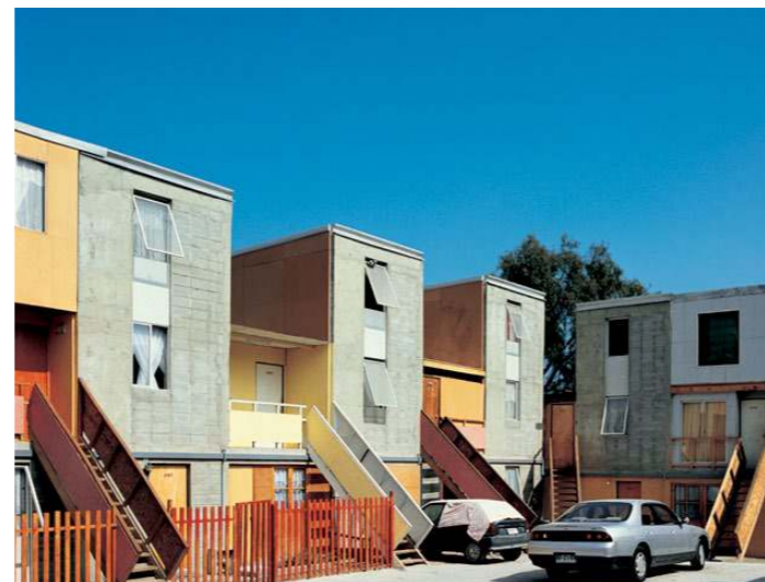
Housing strategy developed for affordable housing in Argentina by A. Aravena where essential infrastructure is built into half of a house with second half for self build.
